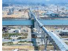
Rikuzentakata recovery embankment (earthquake reconstruction covering 298ha)
