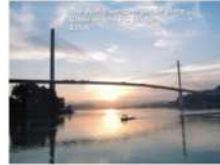
Bai Chay bridge (the longest Single-span cable PC bridge)
