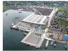
Batangas international container terminal
