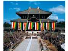
Renovation of the Daibutsuden (Supported with the latest technology)
